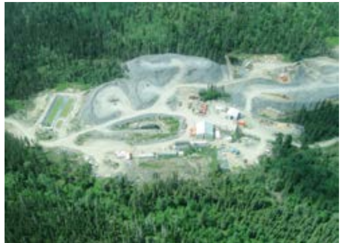
La Ronge gold project's Roy Lloyd mine
