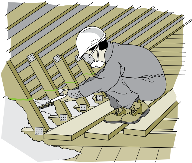
Figure 5-14 Installing loose-fill insulation
