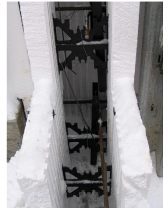
Insulated Concrete Form (ICF)
