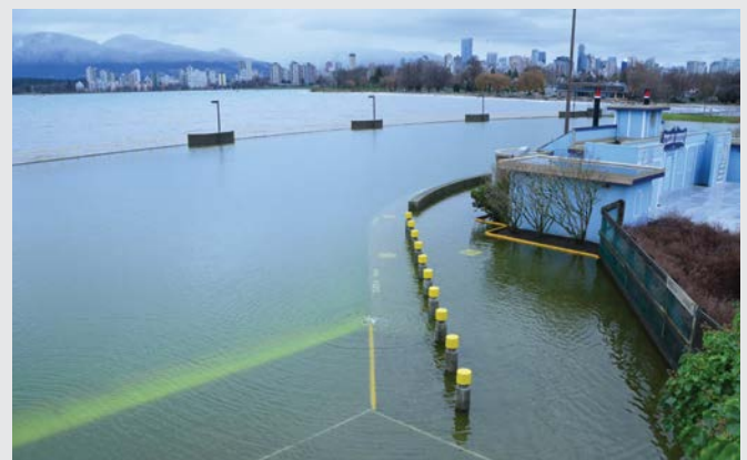
FIGURE 18: King tide of December 17, 2012 with little accompanying wave action caused localized inundation in the City of Vancouver, including flooding of the Kitsilano Pool. Photo courtesy of the City of Vancouver.
