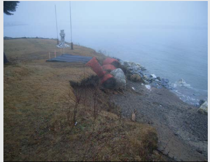
FIGURE 15: Malagawatch Cemetery, NS, where buried human remains eroded into the sea following several storm events. Initial protection of the site involved the use of stone armoring (as seen below the cross). Subsequent storms and erosion led to temporary protection of burials using anchored hay bales and a permeable membrane (centre of photo). Planning for more permanent protection is ongoing. Photo courtesy of Heather MacLeod-Leslie.
