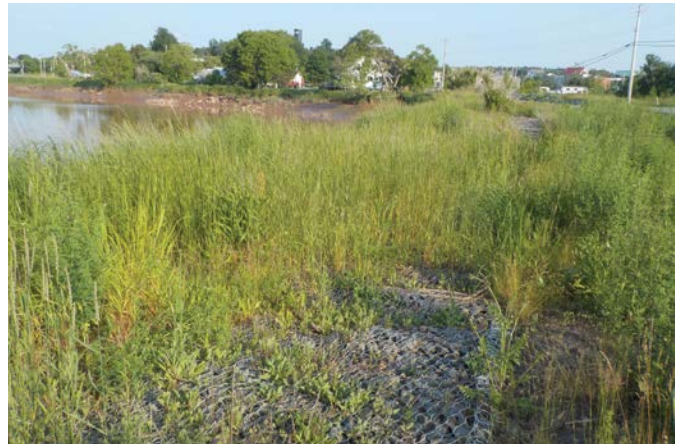
FIGURE 24: Hybrid living shoreline on the Shubenacadie River, Bay of Fundy, NS, illustrating gabion basket planted with marsh vegetation to reduce erosion scour. Photo courtesy of V. Leys, August 2015.
