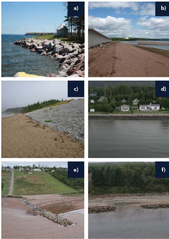
FIGURE 22: Coastal-protection structures commonly used in the East Coast region ( adapted from Jennings et al., 2008 ): a) riprap, Malagawatch ancestral burial grounds, southwestern Bras d’Or Lake, NS (S. O’Carroll, Geo Littoral Consultants); b) seawall, Eel River Bar First Nation, northeastern New Brunswick (D. Bérubé, New Brunswick Department of Energy and Mines); c) revetement, Mispec, southwestern New Brunswick (D. Bérubé, New Brunswick Department of Energy and Mines); d) bulkhead, Maria, Gaspésie, QC (Laboratoire de dynamique et de gestion intégrée des zones côtières–Université du Québec à Rimouski [UQAR]); e) groyne, Paspébiac, Gaspésie, QC (Laboratoire de dynamique et de gestion intégrée des zones côtières–UQAR); and f) breakwater, Pointe-Label, north shore of the St. Lawrence estuary, QC (Laboratoire de dynamique et de gestion intégrée des zones côtières–UQAR).
