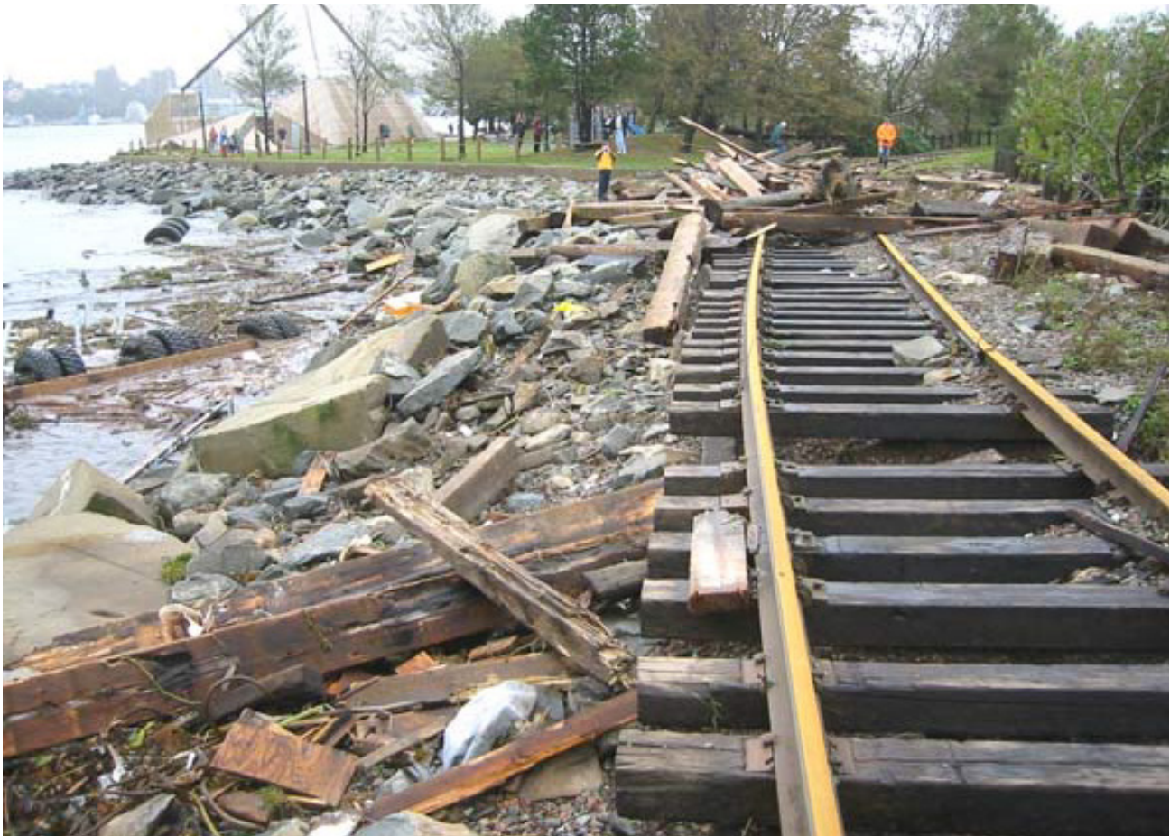
Figure 8: Debris on rail track at Dartmouth Point the morning after Hurricane Juan. Run-up was 1.64 m above the highest water level recorded at the Halifax tide gauge across the harbor, and water levels remained unusually high at the time of photography. (Source: Natural Resources Canada)
