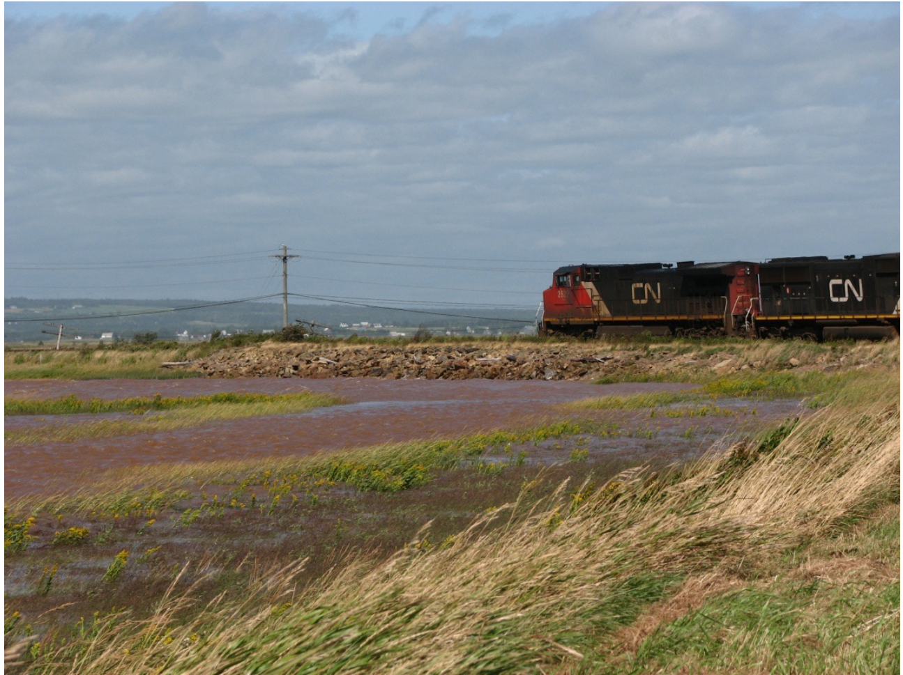
Figure 9: CN Rail in the Chignecto Isthmus. Embankments form part of the region's dyke network. (Source: EOS Eco-Energy Inc.)
