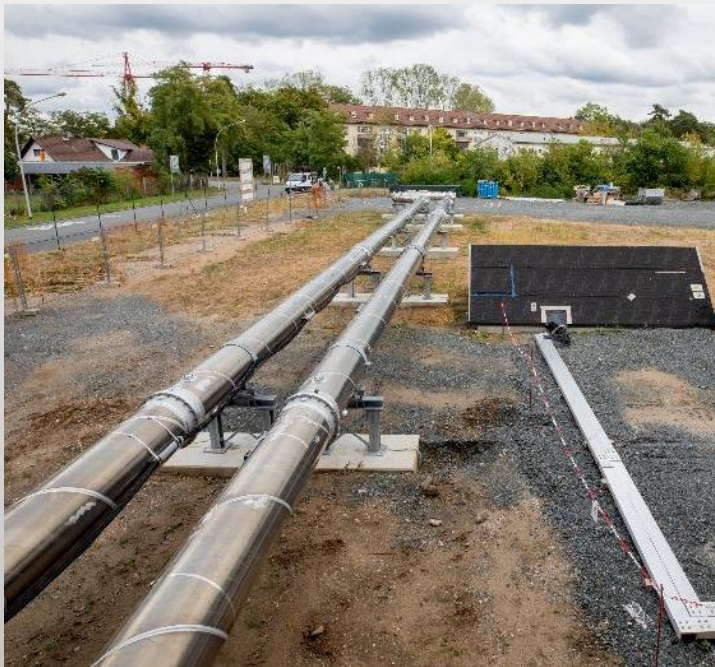
Figure 11: Pilot line (construction phase) for electrical tests; copyright Siemens 40
