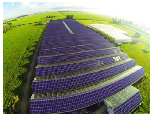
Figure 1: At Vine Fresh Produce Project is the largest rooftop installation in Ontario under the FIT program (2.3 MWp). This project is currently the largest system with Enphase micro-inverter in the world.
