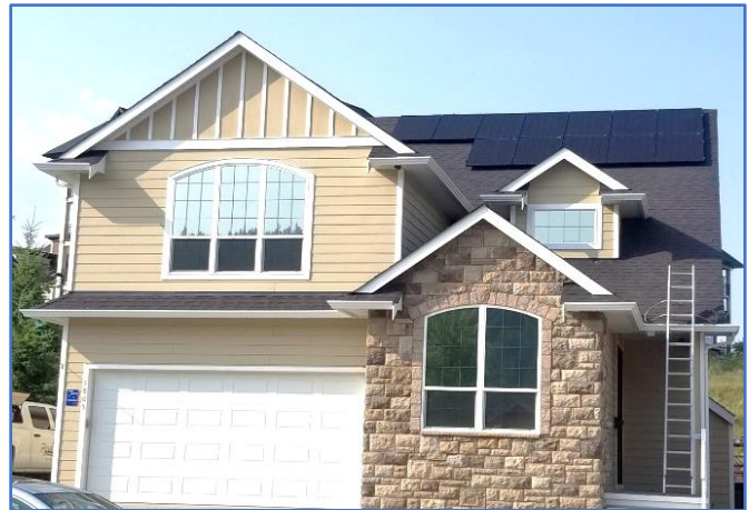
Figure 28: 3.5 kWp Array using Monocrystalline-Cell, All-Black Modules - courtesy Riverside Energy Systems
