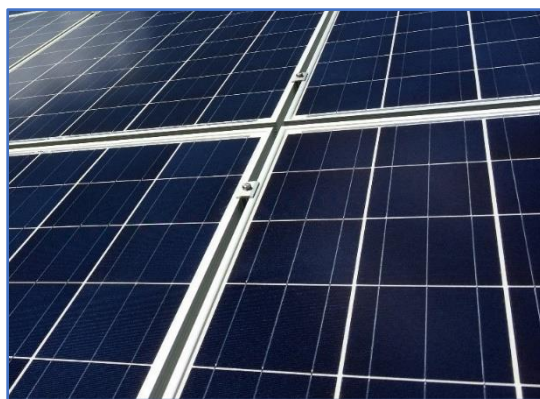
Figure 26: Example of a Polycrystalline-cell module - courtesy of Riverside Energy Systems
