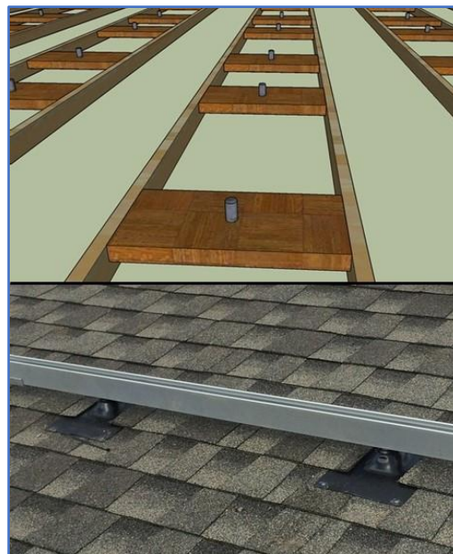
Figure 22: Lag Bolted Anchors to Blocking between Trusses: - Sub-structure (top); Flashed Anchors with Racking (bottom) - courtesy Riverside Energy Systems
