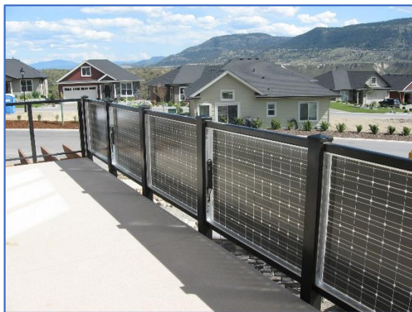
Figure 30: Solar Railing using Bi-Facial Modules - courtesy of Riverside Energy Systems
