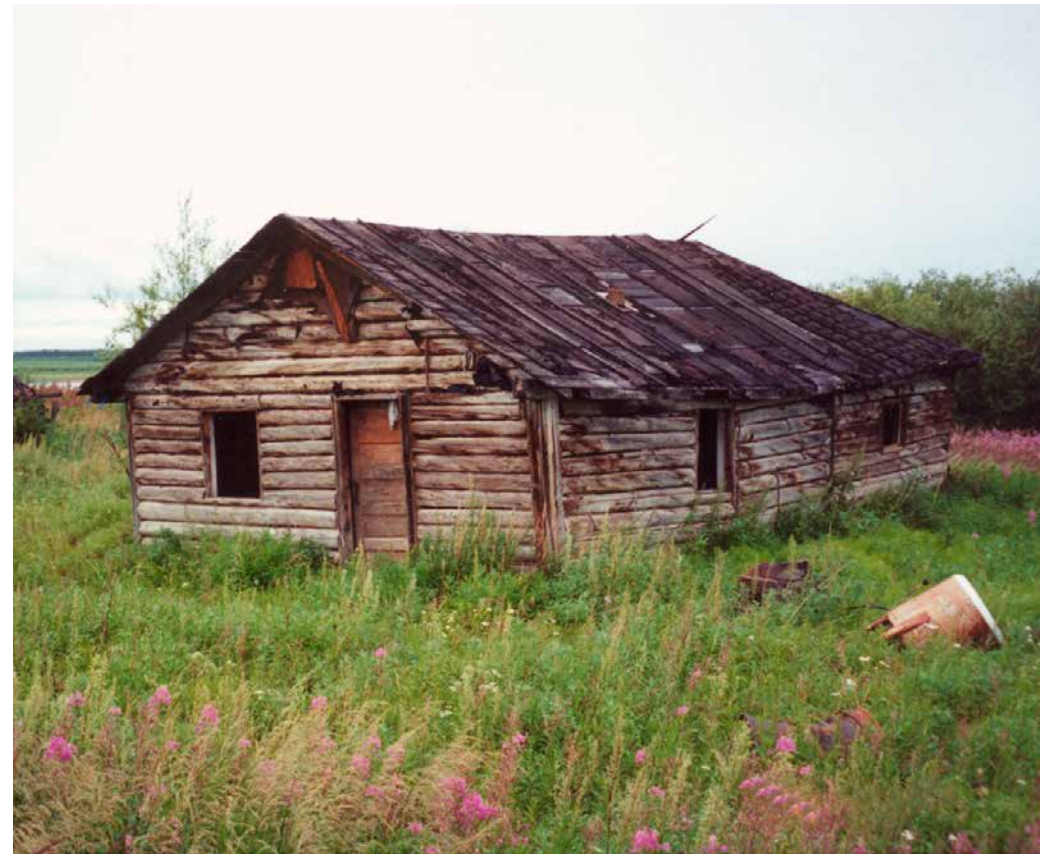
Jimmy and Christie Thompson's cabin, one of many log cabins, warehouses and smokehouses standing at an old village site called Nàgwichootshik (translation: at the mouth of the big country river) near the confluence of the Peel and Mackenzie rivers
