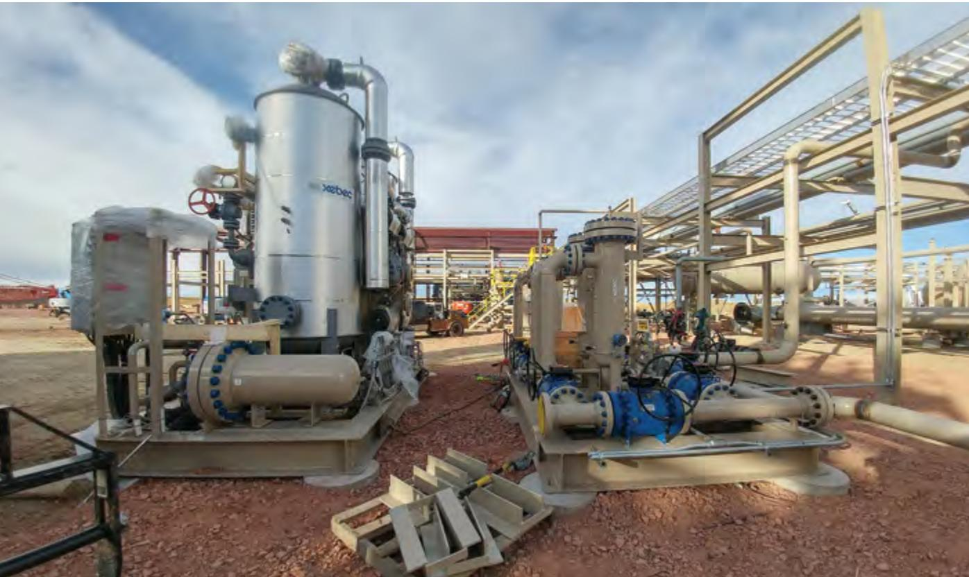
Xebec HRB-type high pressure natural gas dryer for midstream application
