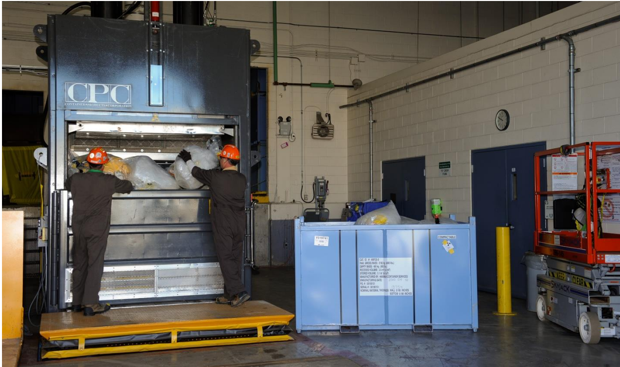
Source: Ontario Power Generation
