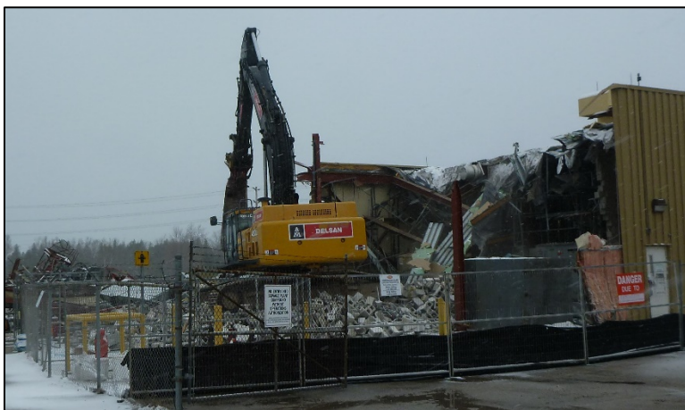
Figure 5: Dismantling of the Spent Solvent Treatment Facility and resulting concrete debris
