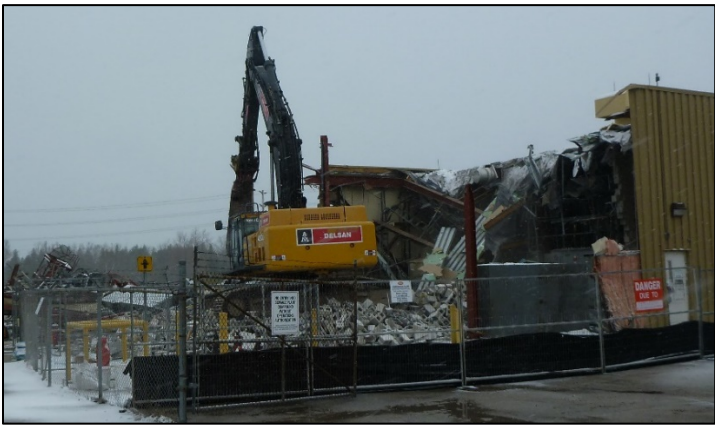
Figure 13: Dismantling of Spent Solvent Treatment Facility and resulting concrete debris
