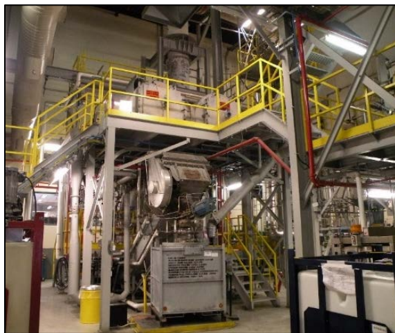
Figure 3: Low-Level Radioactive Waste Incinerator at Western Waste Management Facility
