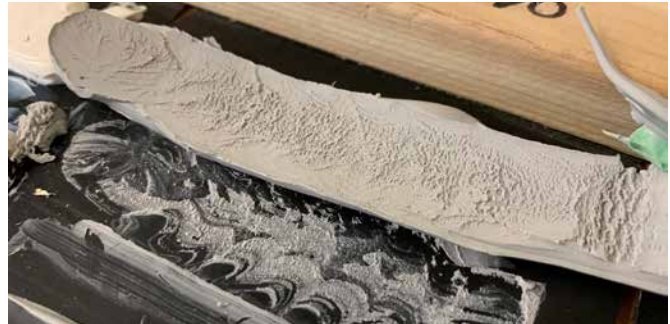
Figure 5 Example of adhesive failure of the sealant bead.
