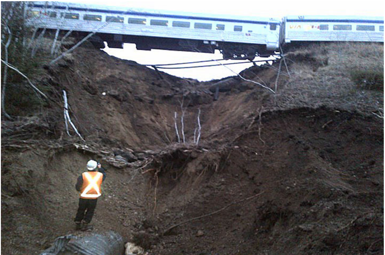
Figure 7: Sub-grade collapse and train derailment due to a frozen culvert in Togo, Saskatchewan, 2013. (Source: Transportation Safety Board of Canada)
