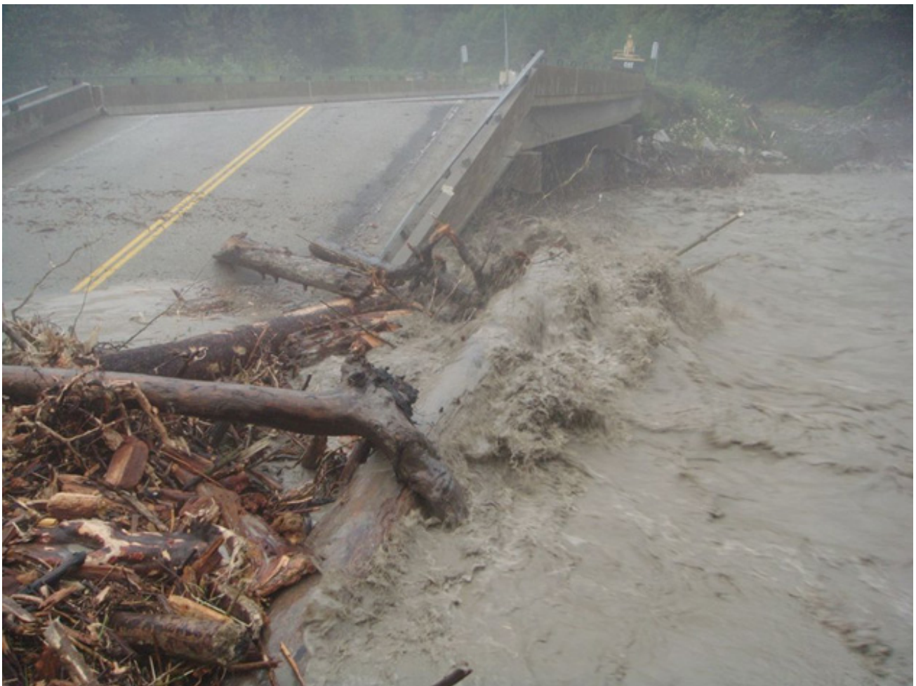
Figure 10: Stewart: Highway 37A Flood Impacts – Bitter Creek bridge failure. (Source: British Columbia Ministry of Transportation and Infrastructure)
