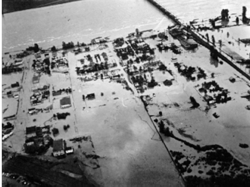
Figure 3: Flood of the Fraser River at Mission, 1948. (Source: Environment and Climate Change Canada)
