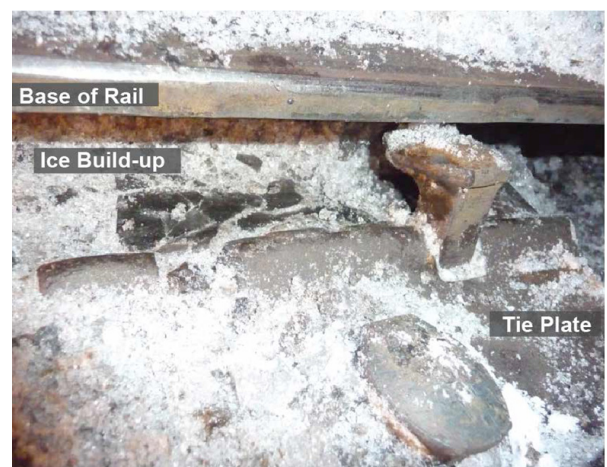
Figure 15: Fernie, British Columbia rail track showing ice build-up. (Source: Transportation Safety Board of Canada)
