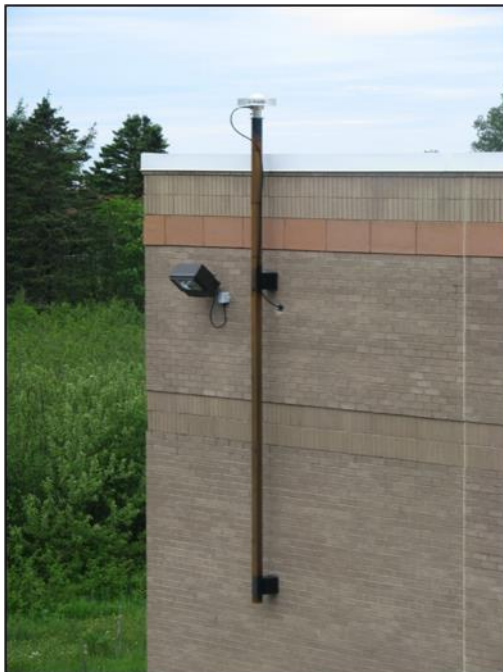
Figure 6 : Antenna mast attached to a load bearing wall
