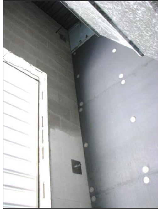
Figure 9 : Through bolts in concrete inner wall
