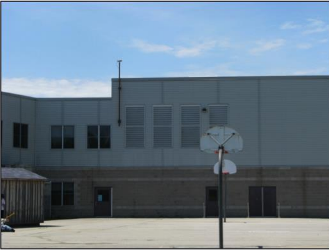
Figure 8 : Metal siding with concrete inner wall installation
