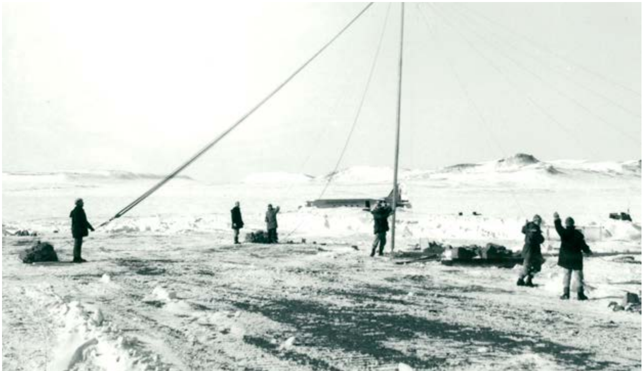
Erecting the transmission mast for the navigation system at the Isachsen weather station on Ellef Ringnes Island in 1959
