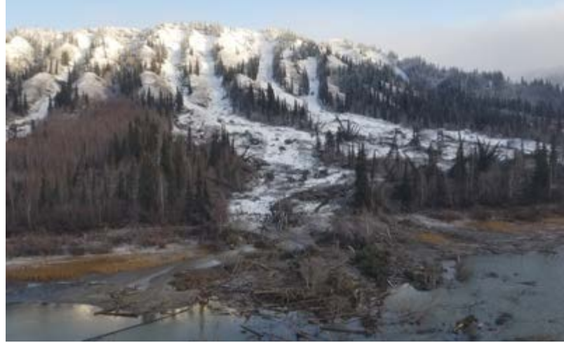
Landslide scars from the autumn 2017 event on the East Channel of the Mackenzie River near Reindeer Station, 40 km north of Inuvik
