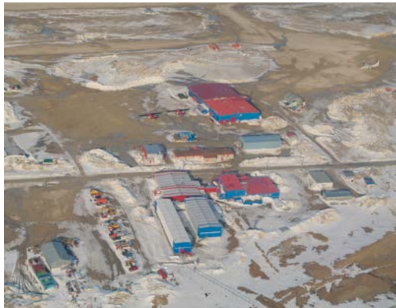
Aerial view of the PCSP facility in Resolute, Nunavut, in 2014
