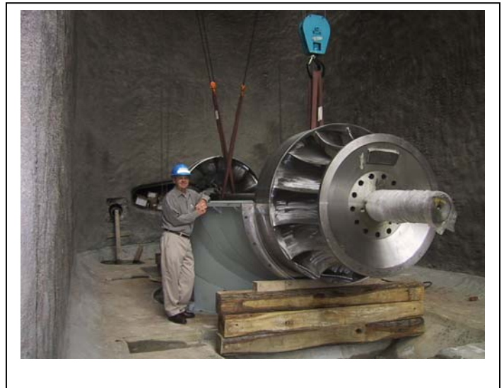
Improved Camelback Francis Turbine in the No. 11 Powerhouse, Energy Ottawa
