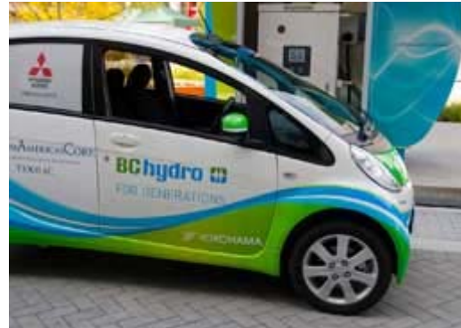
Figure 5: BC Hydro EV charging station. (Source: BC Hydro website)
