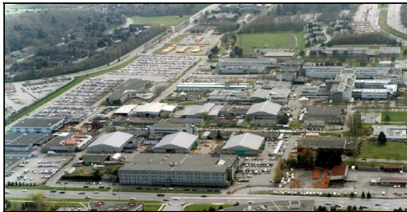
Figure 4: Burnaby Campus of BCIT where smart grid technologies are being demonstrated as part of their microgrid research initiative. (Photo credit BCIT)
