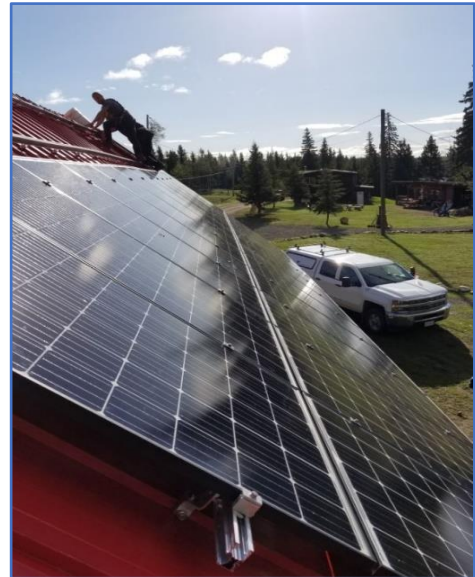
Figure 26: Racking Attachment to Standing Seam Metal Roofing - courtesy Riverside Energy Systems
