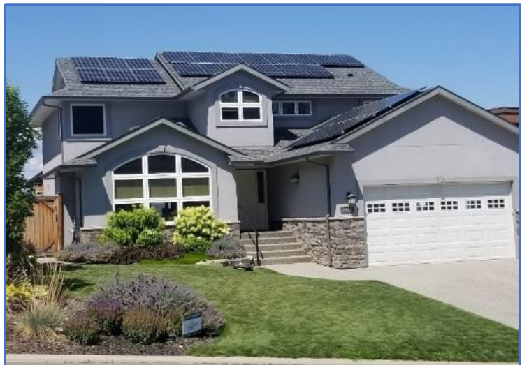
Figure 14: Roof Mounted PV System using South and West Facing Arrays - courtesy Riverside Energy Systems
