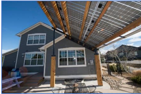
Figure 15: Outdoor Leisure Area Solar PV shelter – courtesy Lumos Solar
