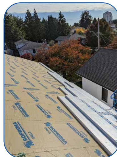
Figure 3 XPS rigid insulation installed over the vapour barrier in preparation for structural cross-strapping.
