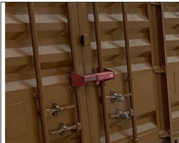
Figure 27 - Example of keeping the vertical keeper bars from turning on a Type-16 magazine
