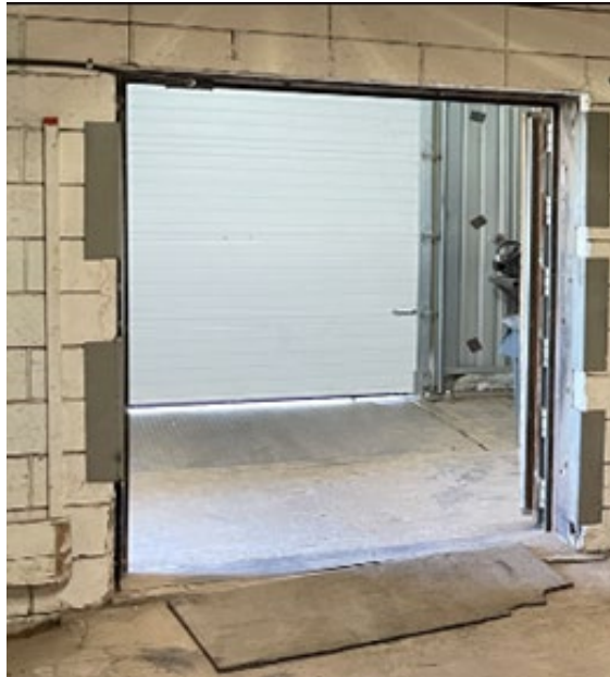
Figure 16 – example of Type-1 magazine door upgraded with steel brackets
