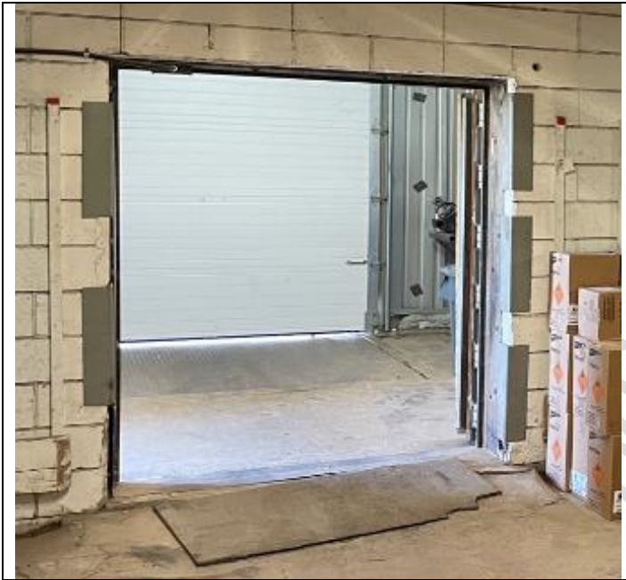
Figure 16 – example of Type-1 magazine door upgraded with steel brackets
